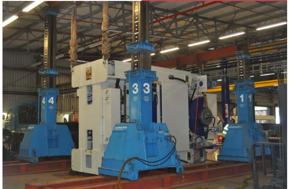
Using Lovemore's Bros hydraulic gantries the steel press is maneuvered into position
